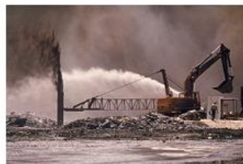
Oil Fire Fighting Companies working in Kuwait 1991 using the displacement tube
