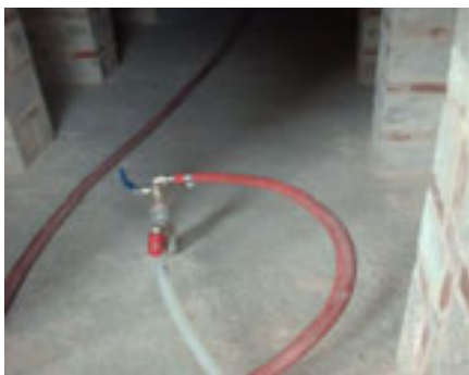
Fig. 3. Supply of the liquid under the foundation
